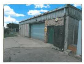
The depot at Stratford Road has a large storage building with a mobile cabin attached as a rest room for the outdoor staff. There are two garages one of which is made of concrete blocks with an asbestos roof and the other of concrete slabs, a composting area, parking for staff cars, a pile of excavated soil from the graves, tree & hedge clippings awaiting disposal and a large skip. The surface of the compound is very uneven.
